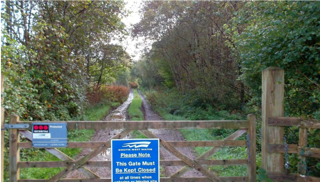
Looking east towards Hatt - the access track to the water treatment plant
