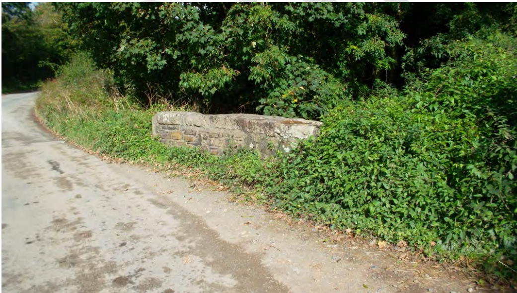
Dean's Bridge - the north parapet
