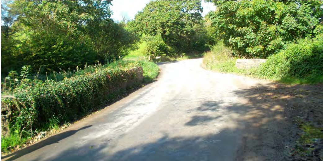
Dean's Bridge - general view
